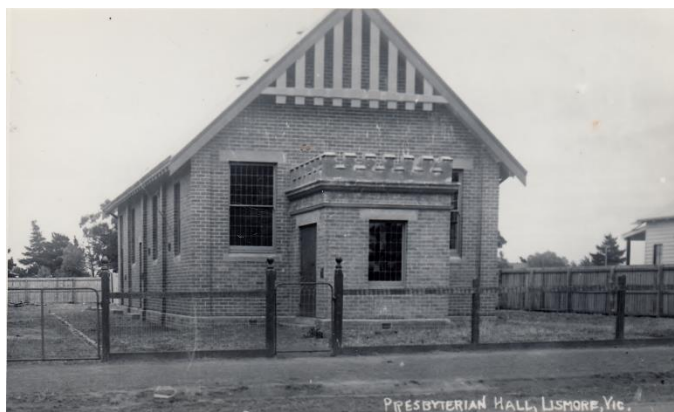
Photo: C1926 soon after erection. JRO_0044
